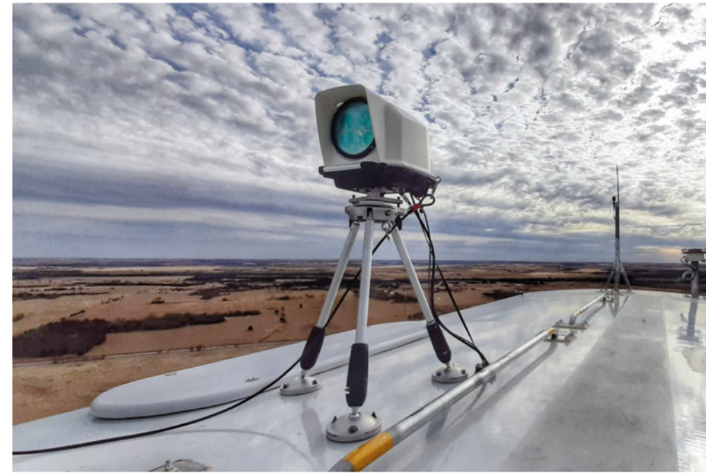
Fig.1 NML installation Photo
