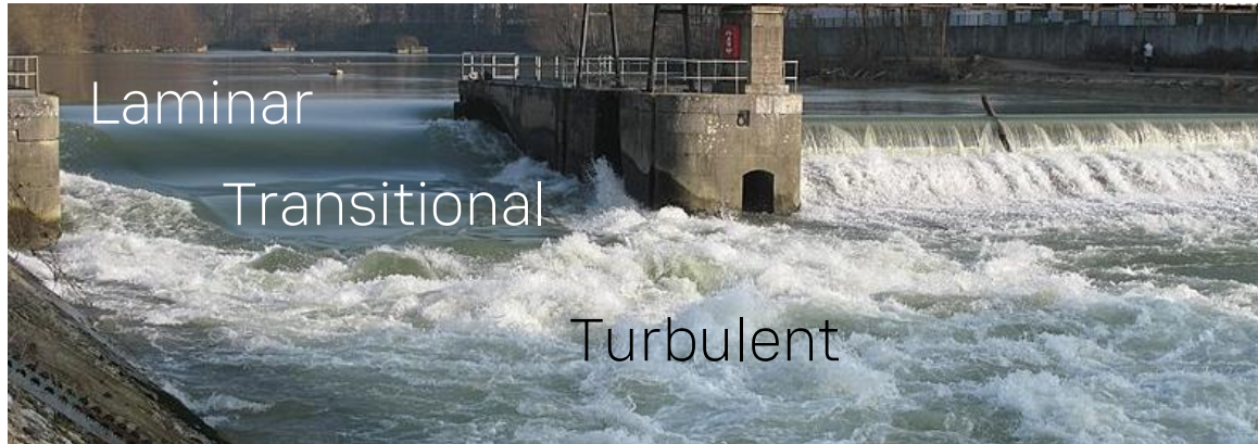
(1) Turbulence in water flow
