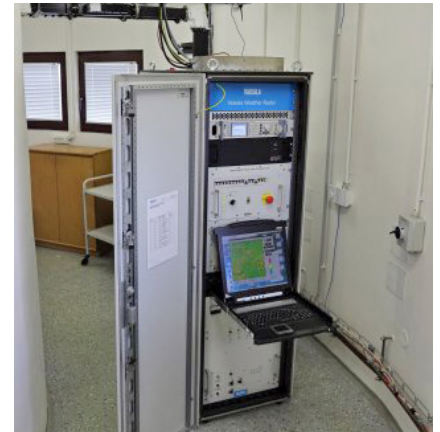
WRM 200 installation at Skalky site
