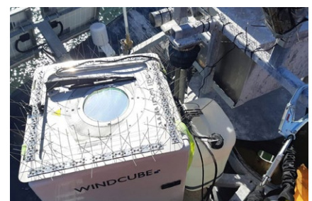
WindCube Offshore on a fixed platform.
