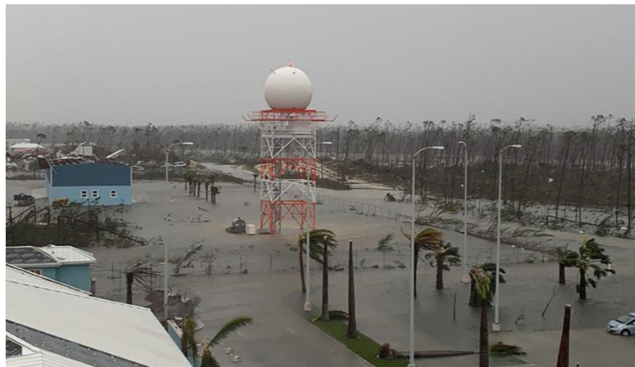
Vaisala Weather Radar at Marsh Harbour Airport in the Bahamas, still standing and measuring after Hurricane Dorian
