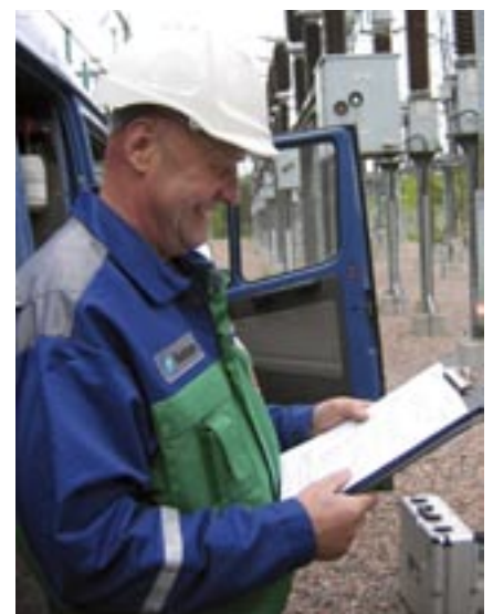
Jussi Penttinen from Fortum Power and Heat makes sure the dewpoint of the SF6 is up to standard at Vantaa Energy's power plant.
