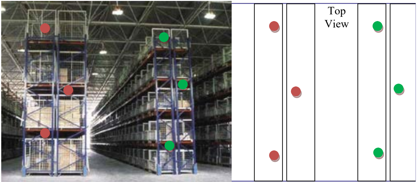
Figure 2: Sensors placed in the middle of racks more closely reflect product temperatures. In this example, nine sensors are located on each double rack in this warehouse measuring 30 meters by 30 meters by 15 meters.
