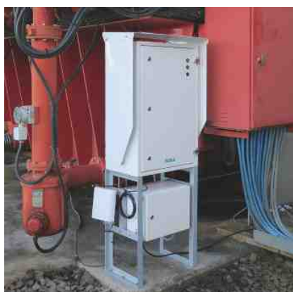
Figure 1. The installed online DGA monitor OPT100. The inlet and outlet oil pipes are connected to the bottom drain valves.
