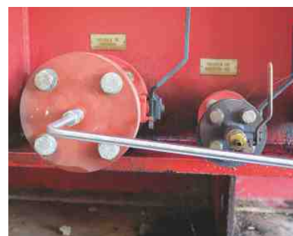
Figure 1. The installed online DGA monitor OPT100. The inlet and outlet oil pipes are connected to the bottom drain valves.
