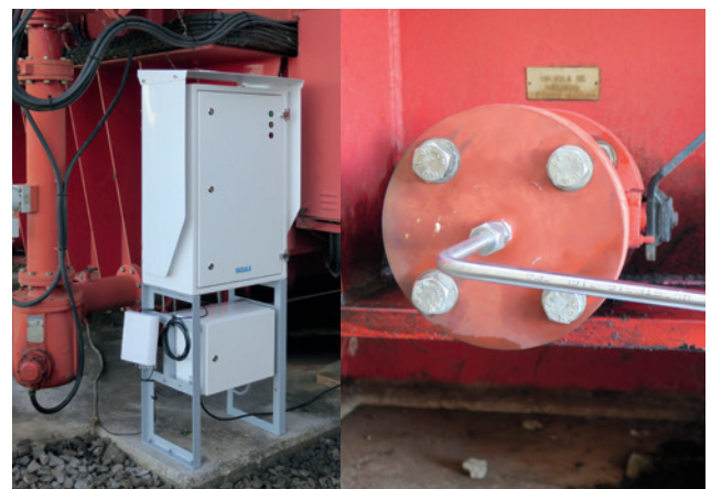
Figure 1. The installed online DGA monitor OPT100. The inlet and outlet oil pipes are connected to the bottom drain valves.
