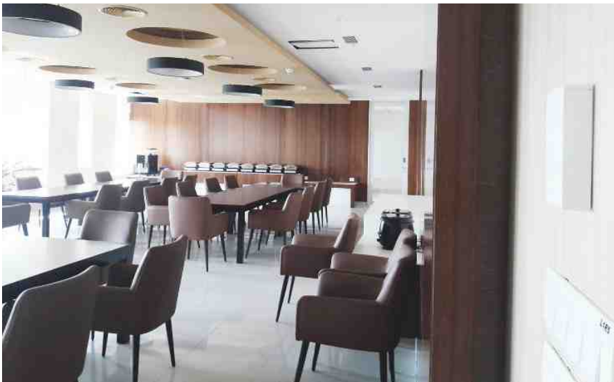
HVAC sensor installation in a dining room in Bangalore campus, Bangalore, India.
