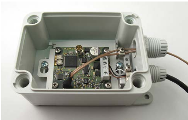
Figure 5 Bracket Installed and Cables Connected
