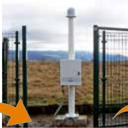
*Sensors instantly detect the electromagnetic signals produced when cloud and cloud-to-ground lightning occurs.*
