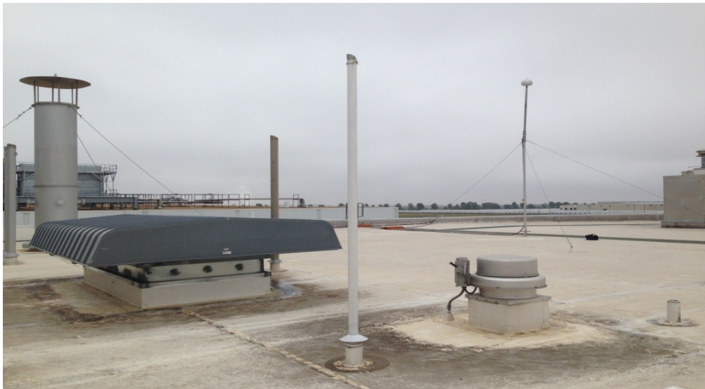
ESE, at right background, competes with other metal objects for air terminal behavior.
