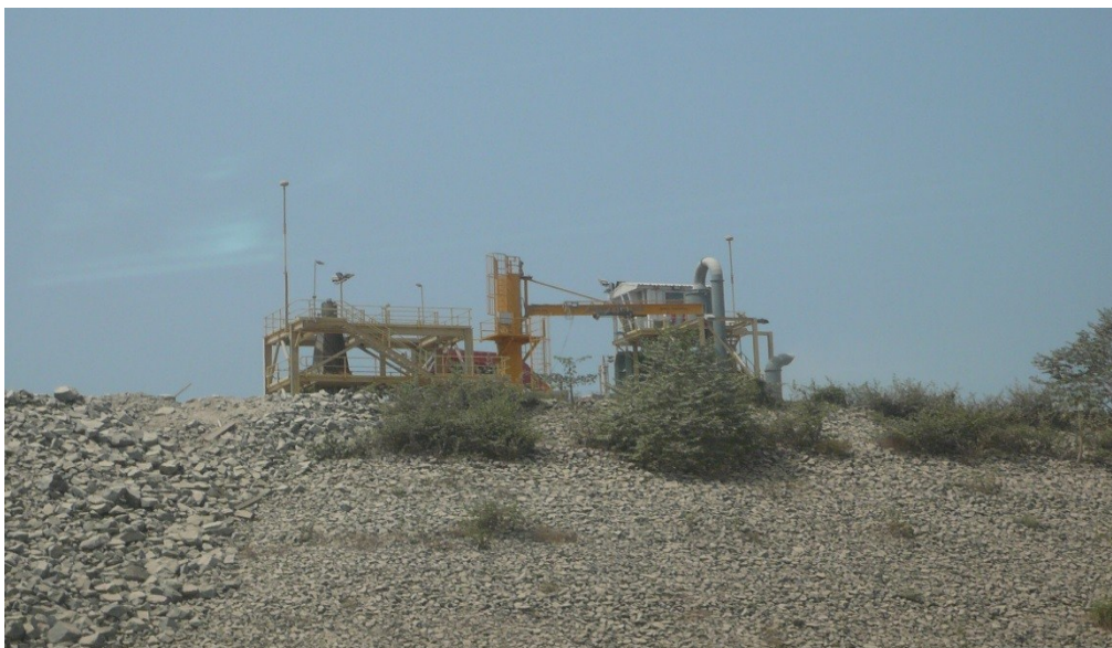
Two ESEs on tall masts. Unnecessary on this all metal structure.
