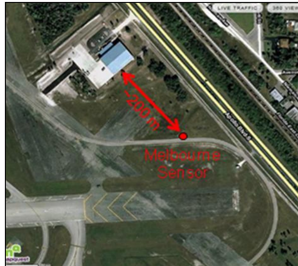
Figure 6. A large metal hanger had been built unknowingly within 200 meters of the cloud-to-ground sensor at the Melbourne airport. This required an update to the configuration settings.
