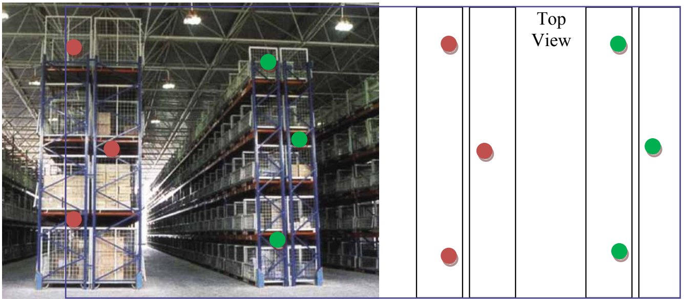
Figure 2. Sensors placed in the middle of racks reflect actual product temperatures. In this example, nine sensors are located on each double rack in this warehouse measuring 30 meters by 30 meters by 15 meters.
