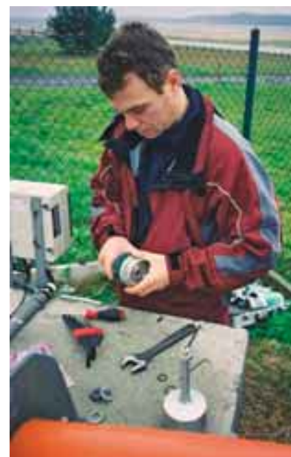
Customer Service Engineer Peter Rowley of Vaisala changes wind sensor bearings and seals.
