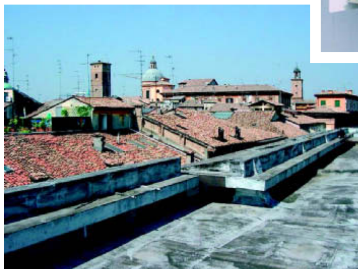
View from Reggio Emilia site. The urban location of the sites required tailor-made system lay-outs to be carried out for each installation site.
