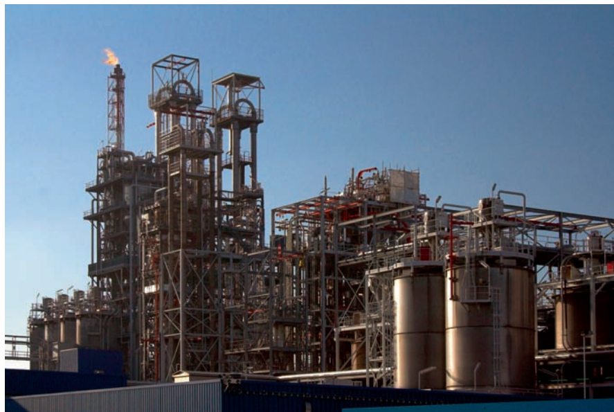
Oxygen measurement is used in ensuring process safety in chemical plants.
