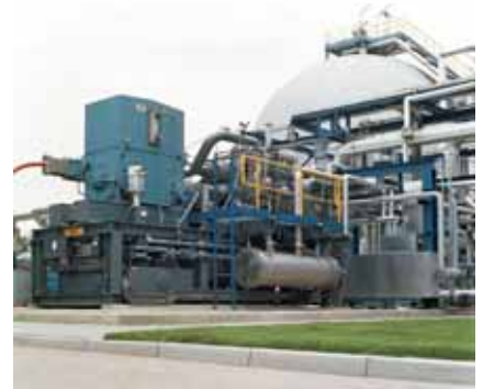
Dewpoint monitoring of compressed air.
