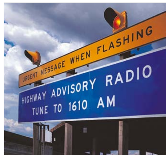
Message signs alert motorists to tune their radios to the right frequency.
