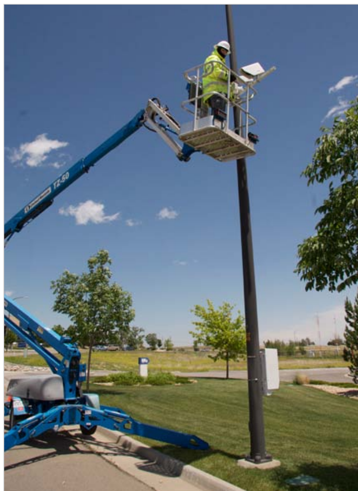
Vaisala Guardian can be quickly and easily mounted on existing structures above or beside the road. Non-invasive installation also means that the system can be easily relocated whenever necessary.
