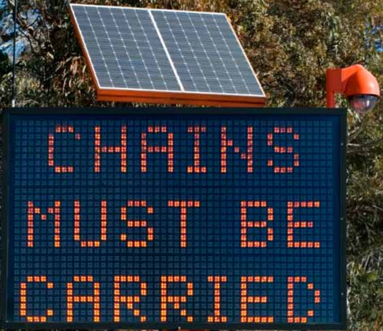
Portable electronic message signs enable flexible ways for communicating information to drivers.
