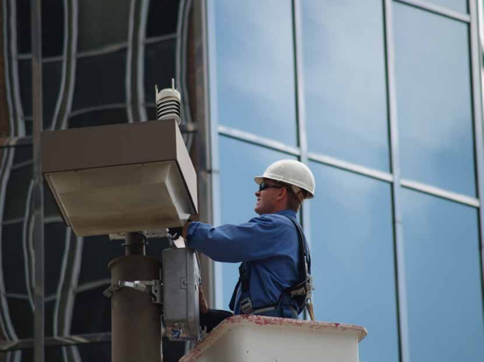
A Micronet technician deploys a traffic light station on 8 May 2008. The Vaisala Weather Transmitter WXT510 is a key component of the Oklahoma City Micronet.
