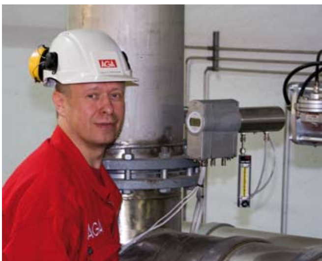
Heimo Märkälä demonstrating the OMT355 installed at the AGA Kaukas plant.
