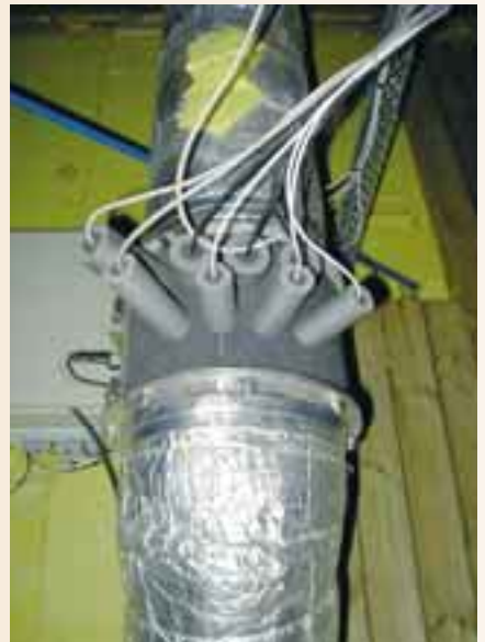
The lead-in holes of the sensors were insulated.
