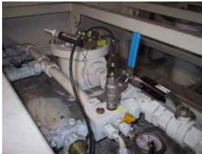
A HMP228 unit installed in a ship's machine room. Installation is easy and convenient to perform through a ball valve.
