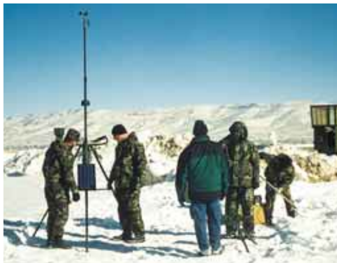
TMOS being installed at Mountain Airport. Note mobile ATC Tower on Humvee in the background. TMOS hard-wired to PC in ATC Tower for airport operations. Temperature at the time is -4 °F (-20 °C).
