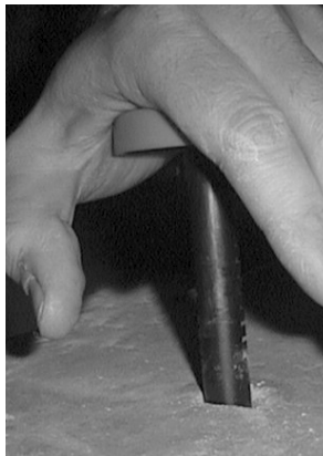
Figure 5.1 Pressing the sleeve into the hole
