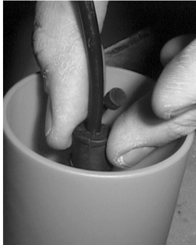
Figure 5.3 Sealing the sleeve with a plastic plug
